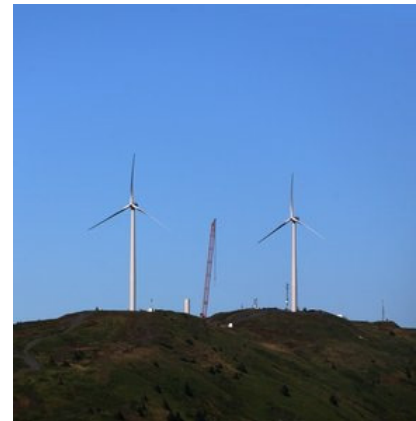
Each of these turbines produces up to 1.5 MW of electricity
