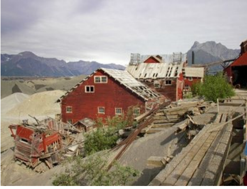
Kennecott Leach and Flotation Facility
